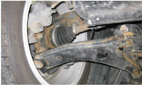
Fig. 1 Chassis Condition after Car Corrosion Test
