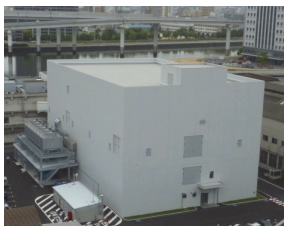
Fig. 1 View of New Climate Testing Laboratory
